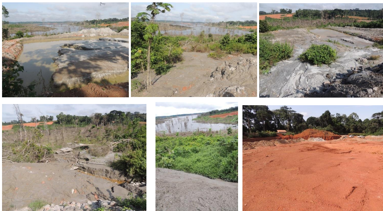
Figure 2-3: Bassins de sédimentation
