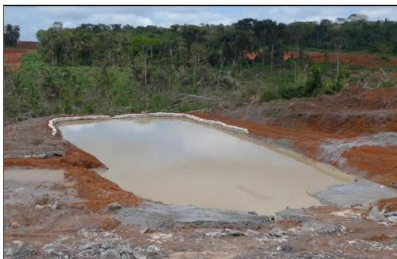
NOUVEAU BASSIN DE SEDIMENTATION CONCASSEUR 200T, TROP RAPIDEMENT SATURE (PLEIN DE SEDIMENTS)
