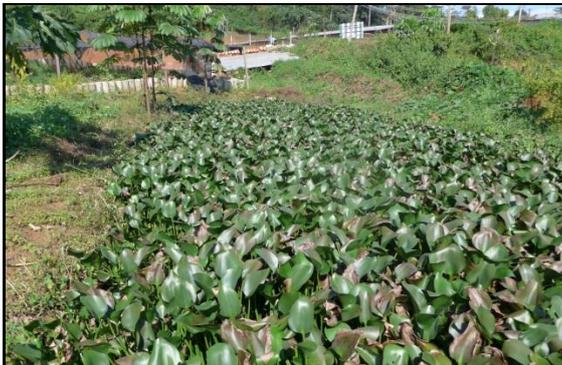
BVC : LE BASSIN D'OXYDATION RECOUVERT DE JACINTHE D'EAU DOIT ETRE FAUCARDE
