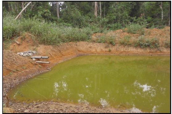
PAS DE LIXIVIATS PRODUITS EN SAISON SECHE. L'EFFLUENT DU BASSIN D'OXYDATION EST CONFORME EN DBO5.
