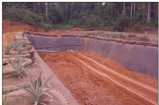
*...ET EN FEVRIER: DEPOT EXCESSIF DE TERRE QUI REDUIT LA DUREE DE VIE DE LA CELLULE*
