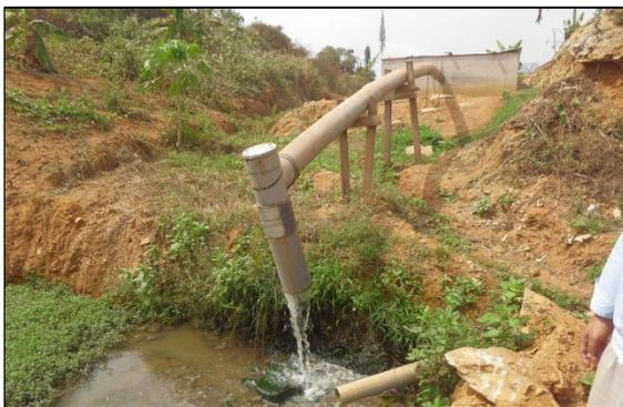
*BVO TOILETTES ET DOUCHES: SORTIE DES FOSSES SEPTIQUES ET ARRIVEE DANS LE BASSIN D'OXYDATION.*
