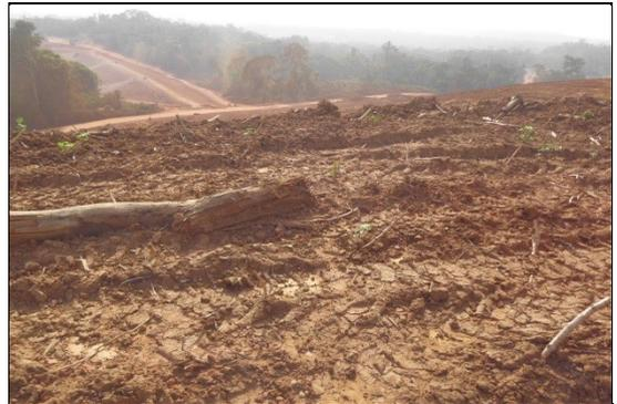
TERRE VEGETALE EN COURS D'EPANDAGE SUR LE PLATEAU DU DEPOT 4. AUCUN DRAINAGE PERIPHERIQUE.
