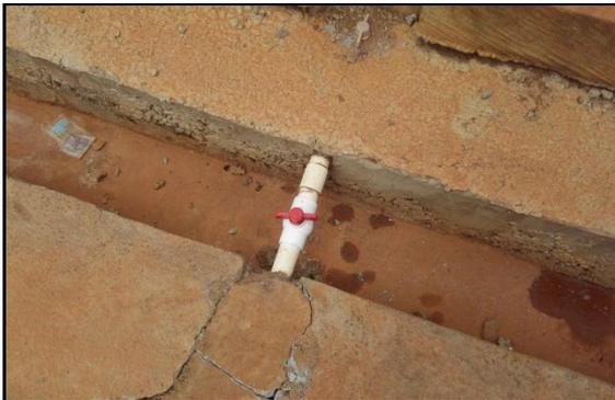
DEPOT PRINCIPAL DE CARBURANT : VANNE D'ACCES DESHUILEUR EN POSITION FERMEE : CONFORME
