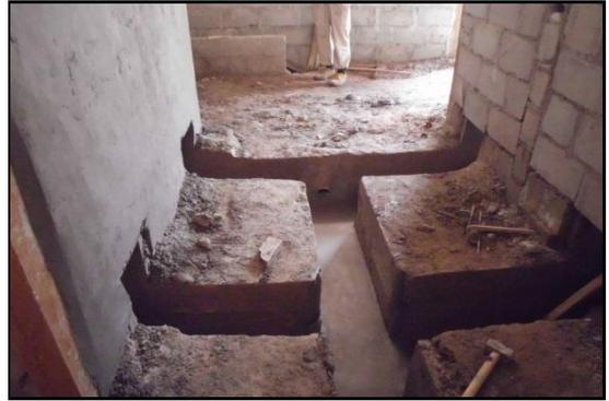
LA JONCTION DES 4 CANAUX N'EST PAS HYDRAULIQUEMENT APPROPRIÉE ET NE FONCTIONNERA PAS CORRECTEMENT
