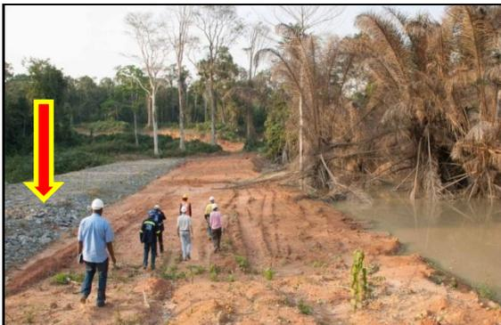
BASSIN DE SEDIMENTATION SOUS CONCASSEUR : LA DIGUE (FLECHE) DOIT ETRE REHAUSSEE DE 2 M
