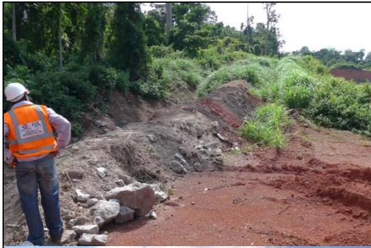
MERLON DE PROTECTION REALISE SUR LA TOTALITE DU PERIMETRE DE LA CARRIERE
