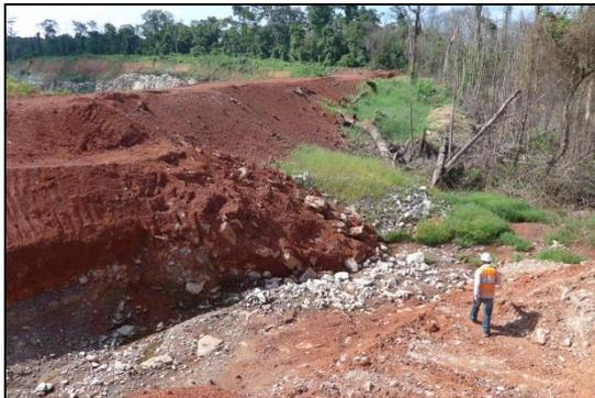
SECONDE TRANCHEE DANS LA DIGUE PERMETTANT L'ECOULEMENT DES EAUX DU BASSIN VERSANT
